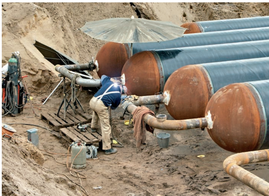
Fig. 2: Welding work on the small-bore piping
