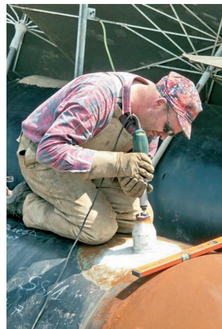
Fig. 3: Work on the venting sockets
